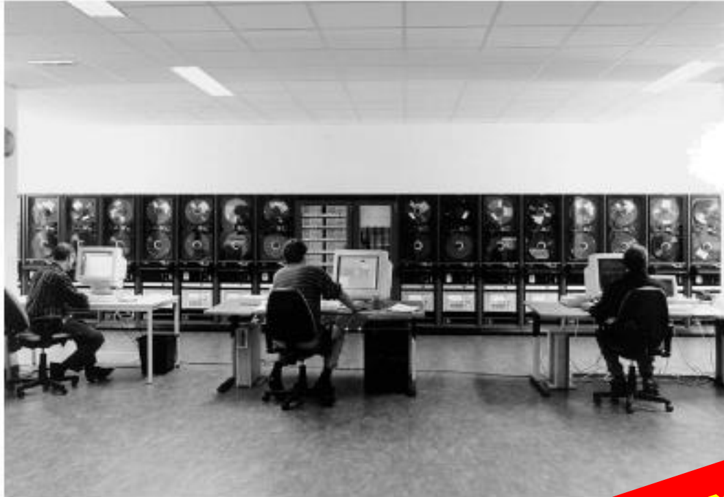
The JIVE Data Processor control room. The row of 16 DPUs
