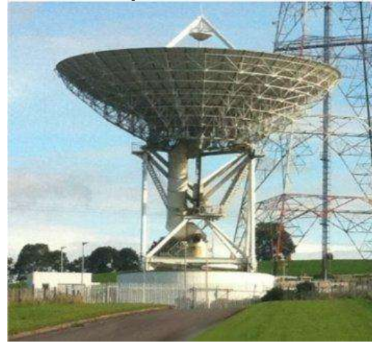
Ireland Elfordstown – handed over 2011/05
