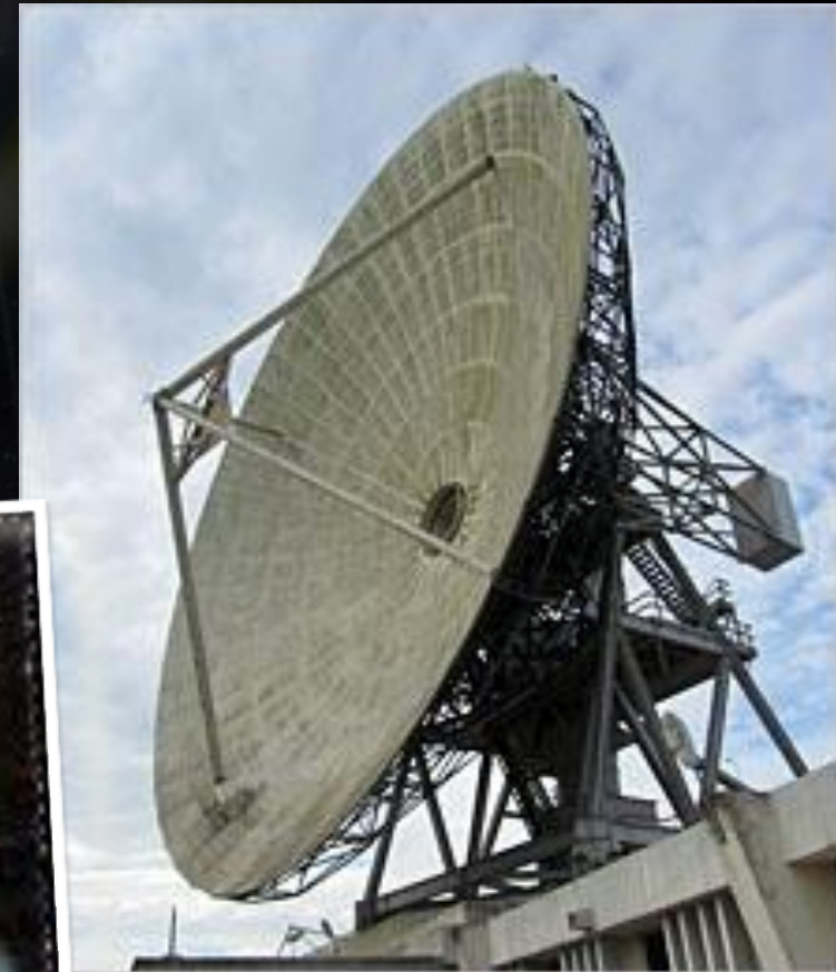
Ghana's 32-m satellite communications antenna
